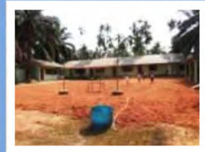
New Front Wall and dirt for playing area.
